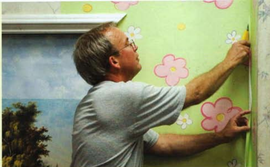
Rickrode trims wallpaper to demonstrate how to properly paper a corner during a seminar at York Wallcoverings.
